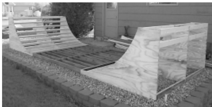
Frames put together before attaching the decking.
